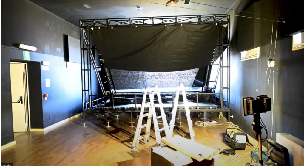
Fig. 2. Holotheater under construction in the fourth room of the Astrolab. The truss structure supporting the foil can be seen, as well as the horizontal suspended structure that holds the LED wall, which was already installed in the photo. The overall size of the entire structure is clearly perceptible.
